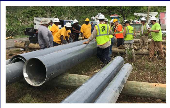
WAPA and BBC Electric crews work on composite pole assembly.
