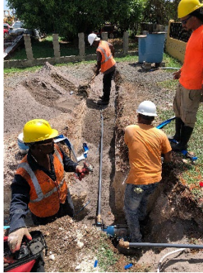
Figure 1: WAPA's Water Distribution Department working to replace outdated piping infrastructure.
