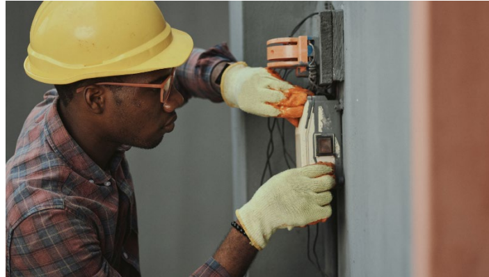
Figure 1: Electrician performing field work. (Stock Image)
