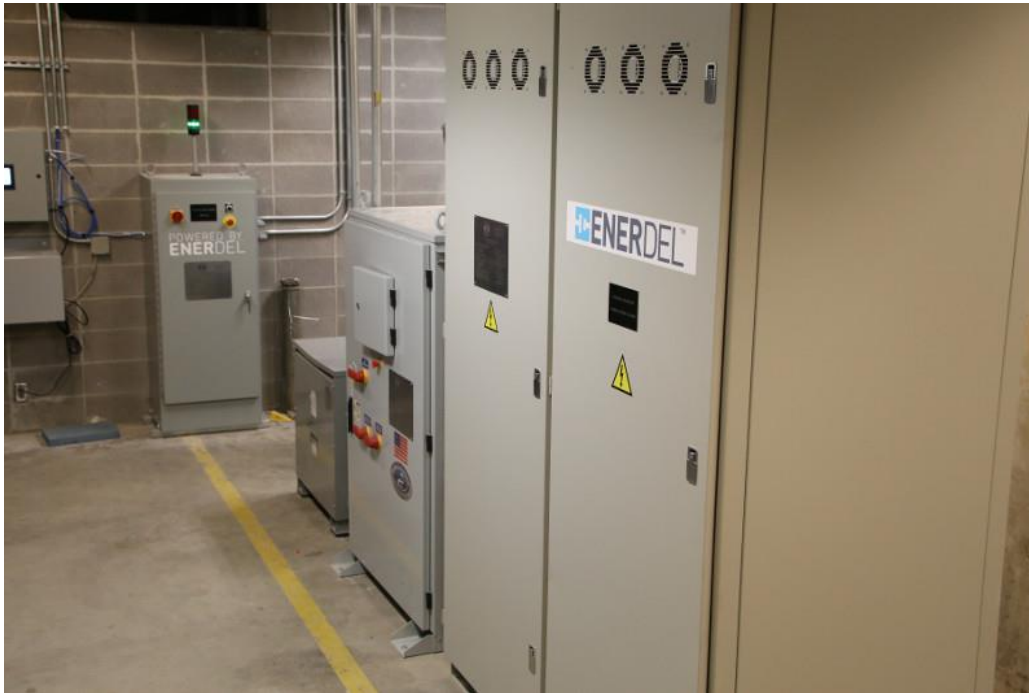
Figure 4-3 Lithium Ion Battery Energy Storage System Located at the Black & Veatch Headquarters
