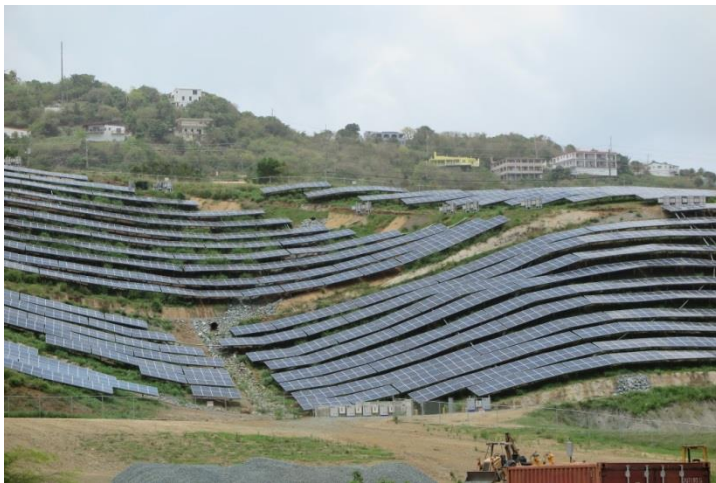
Figure 4-1 USVI Solar I Project Site (Complex Terrain)
